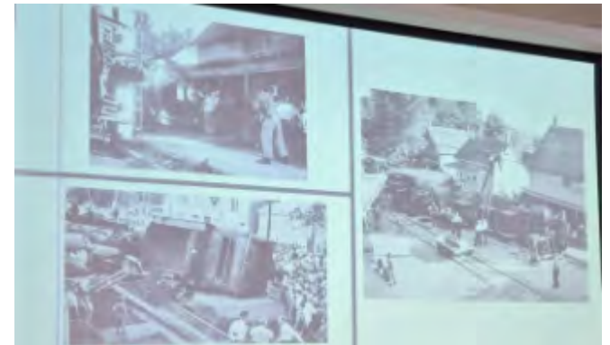
Hazards of street railways; a runaway on steep street and a sharp curve at the bottom put a CP switcher on her side
