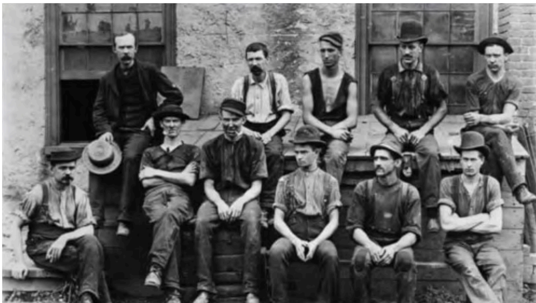
Figure 5-15 A circa 1900 work crew with the boss man in the upper left. Photo courtesy of CNBC – photographer is unknown.
