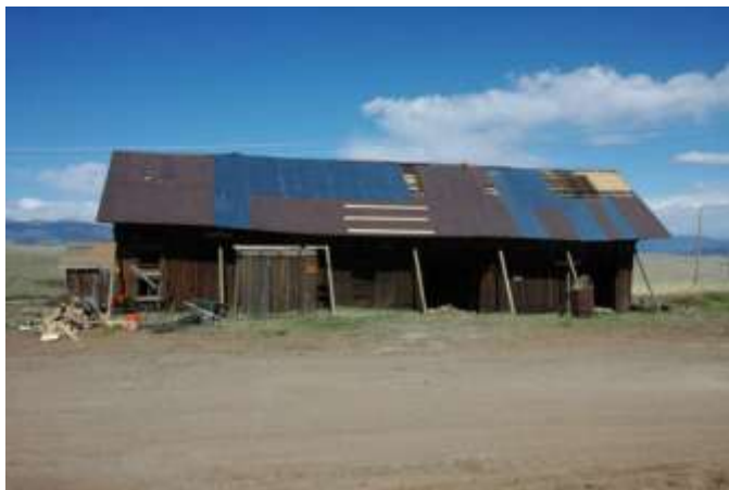
Photo 3: (Center) - Stabilization June 2008 (Now under new ownership and designated as a historical building, the Colorado Preservation Inc. stabilizes the leaning walls)
