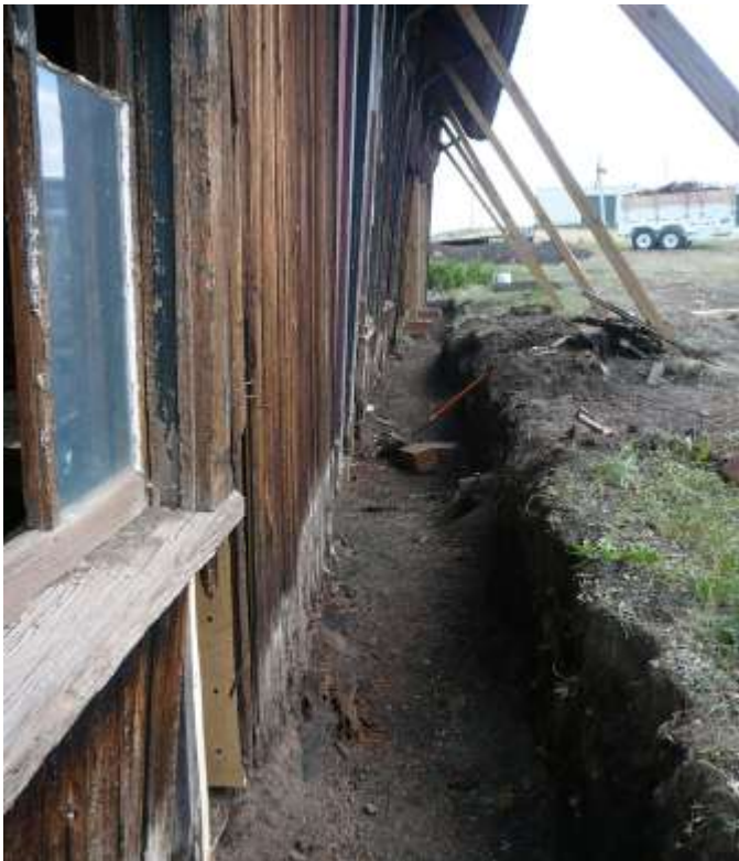
Photo 4 Trench dug along front wall to find the buried footings.
