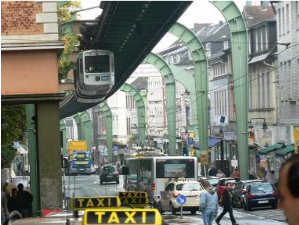
A view of Vohwinkel, near the western terminus of the suspended monorail. The rail is suspended at a height of 8 m or more to allow for clearance for street traffic below.
