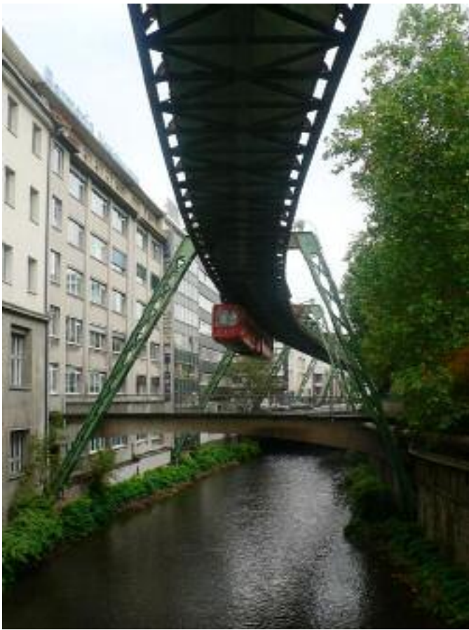
A train on the suspended monorail in the center of Wuppertal.
