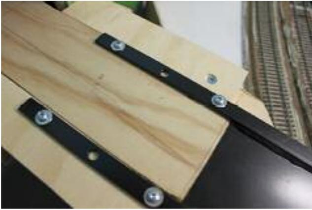
Photo 3: The right hand end of the bridge is held on place with #6 screws and washers through over sized holes.
