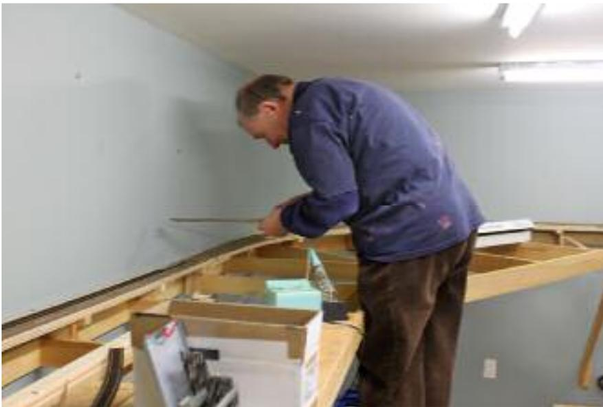
The Photo on the left shows David Steer busy installing the flex track on top of the cork. We are experimenting with a new fastening approach where the track is set in a thin bed of silicon sealant. So far this approach is working out very well though it does require careful cutting and pre-bending of the track before gluing in place.
